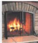
Properly Screened Woodburning Fireplace
